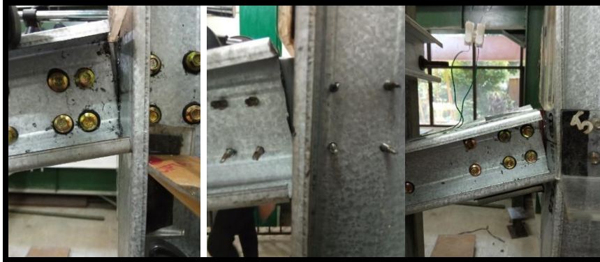
Figure 4.11. Failure of the Gusset-Plate Screw Connection
