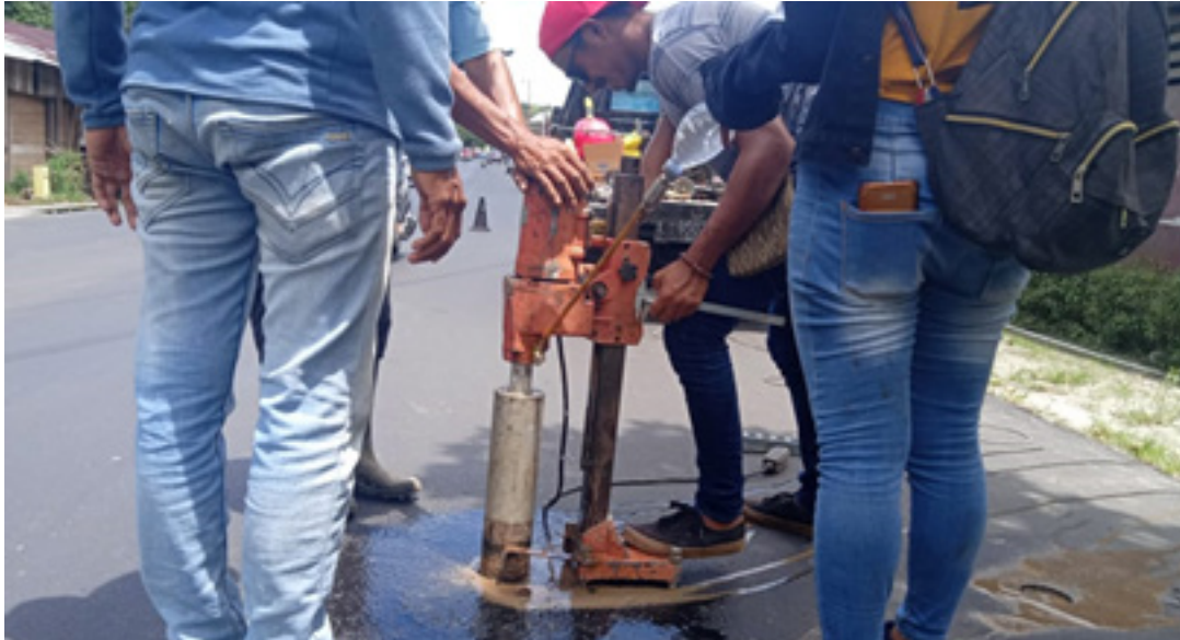
Gambar 9. Core drill Sta. 1+900 (R) Jalan Leo Wattimena
